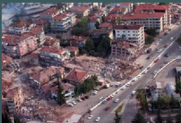
Figure 2: A general view of building damage in Golcuk
